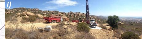
i) This panoramic photo shows the installation of RD-120, which was installed to evaluate flow paths that could be transporting TCE or its daughter products from the Canyon RFI site along the Happy Valley Fault zone. An old road had to be restored to gain access to the drill site. Rock core and groundwater samples from this well show no TCE or daughter product impacts.
