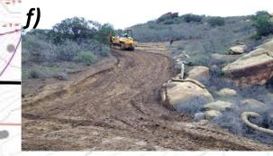
f) Roads had to be restored to access certain locations for well installation. Cultural and biological surveys were conducted prior to cutting the road to the drill site. This road leads to the location of a well drilled to characterize potential source inputs from the Instrument and Equipment Laboratory RFI site. Groundwater samples were collected in February and results are pending.
