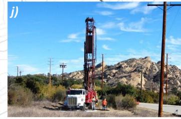
j) Care must be exercised when installing wells near overhead power lines as minimum "Stand-off" distances are needed to prevent arcing of electrical current from the power lines to the drill rig's mast.
