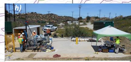
h) A new drilling method was attempted to characterize historical releases to groundwater at the Advanced Propulsion Test Facility RFI site. The "Hydracore" rock coring method results are being compared to standard rock coring methods. Results of the comparison are pending.
